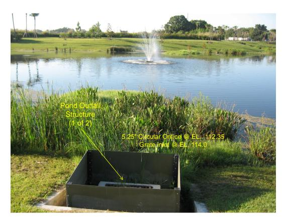
Figure 1-8. Outfall Structure for the Pioneer Key Pond.
