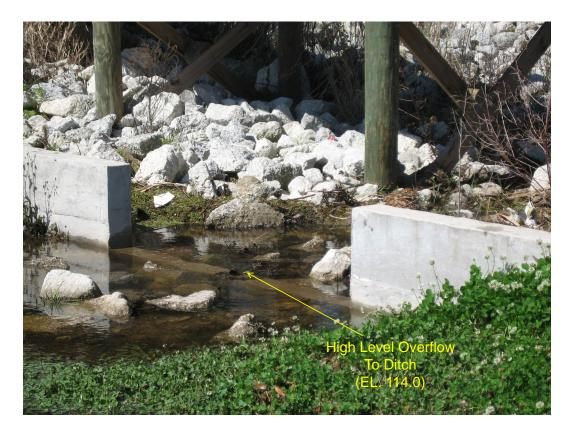
Figure 1-9. High Level Overflow Structure on the Northeast Corner of the Pioneer Key Pond.
