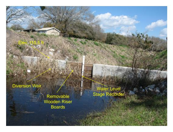
Figure 1-5. Diversion Weir Structure in the Northwest Ditch.
